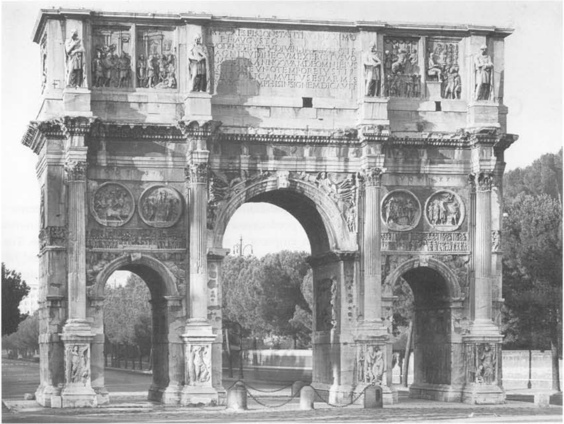
FIG. 1 – Rome, Arch of Constantine, northern facade (photo: Deutsches Archäologisches Institut Rom, neg. 61-2297).
